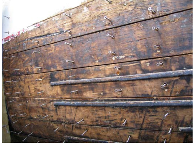
Screws in place ready for driving
