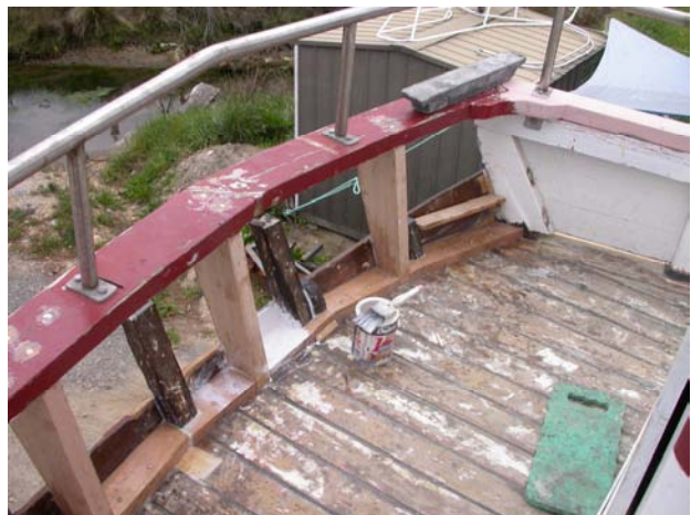
Deck sealing and new stanchions
