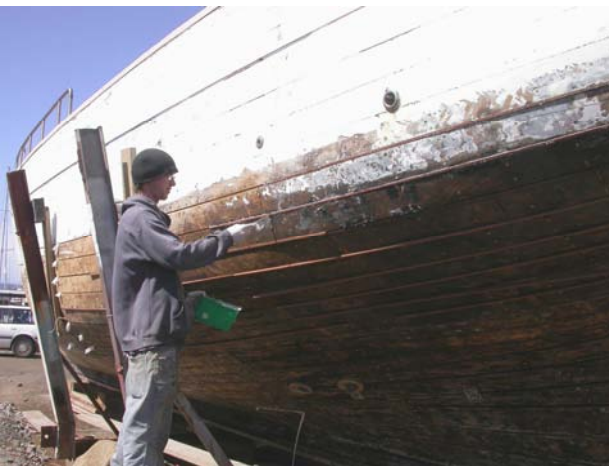
Mick Perigo gluing in splining strips
