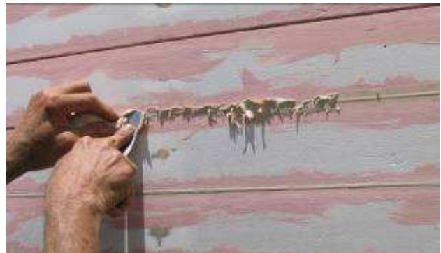
Pressing putty into the seams on top of the caulking.
