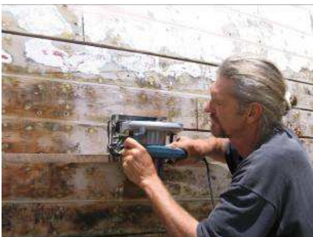
Cutting grooves between planks with a circular saw
