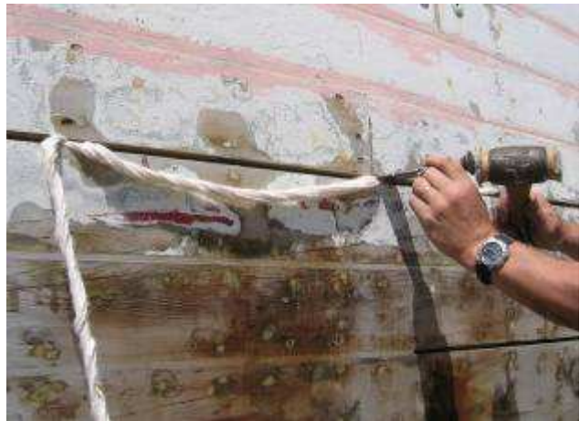
Hammering in the caulking cotton
